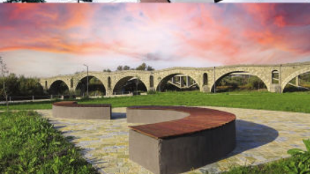
Fig. 23 Tabakëve Bridge - An iconic bridge 127 meters long and 4.03 meters wide, built in the 17th century with carved stone over the Erenik River.
